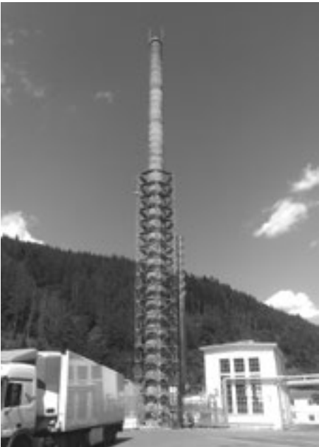
➤ p. 281 DEMOLITION OF ORIGINAL 65-METRE CHIMNEY.
