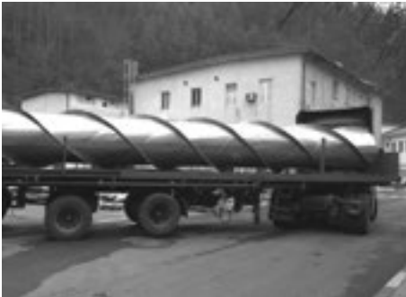
➤ p. 281 DELIVERY OF THE MAIN BODY OF THE NEW CHIMNEY.
