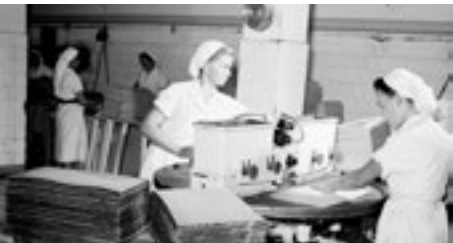
➤ p. 109 WAFFER PRODUCTION – AN ELECTRIC OVEN FOR THE WAFFERS – A WORKER TAKING OUT THE COOKED WAFFERS FROM THE BAKING PLATES AND SPREADING THEM.
