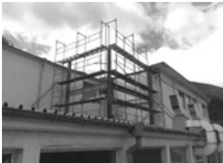
➤ p. 273 MASS LINE 'TOWER' UNDER CONSTRUCTION.
