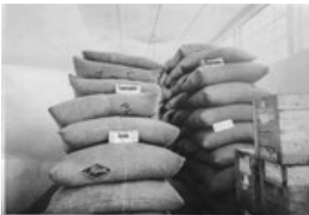
⌘ p. 47 FOURTH FLOOR OF THE ISKRA FACTORY IN SVOGE (TODAY'S LINE FOR MANUAL ARRANGEMENT OF PRALINES – PL16), A WAREHOUSE FOR RAW CACAO IN SACKS WITH THE PEEV LOGO AND SIGNS WITH THE ORIGIN OF THE CACAO ARE VISIBLE.
